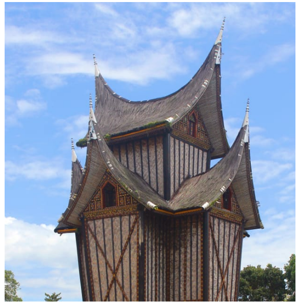
Figure 3. the gonjong roof of the rangkiang building in the courtyard of Pagaruyuang Palace (Author's Document, 2017)
